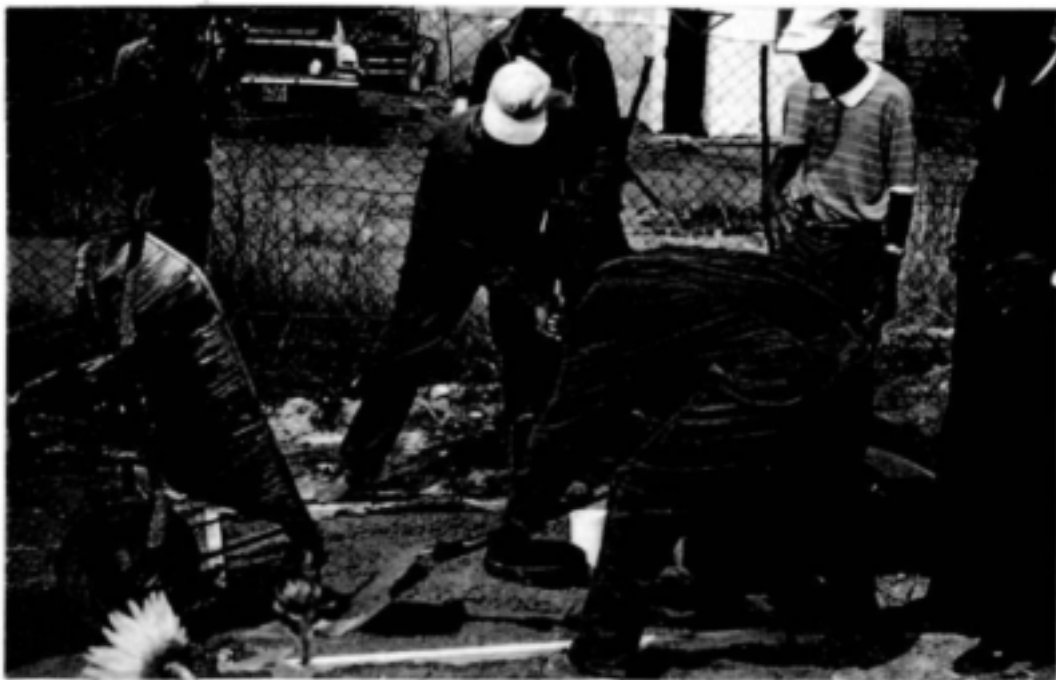
Photograph B : Casting of concrete floor slab
