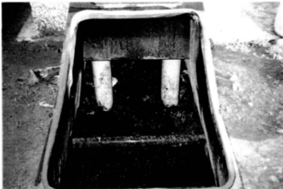
Photograph N : Flooded latrine container as a result of incorrect wastewater disposal
