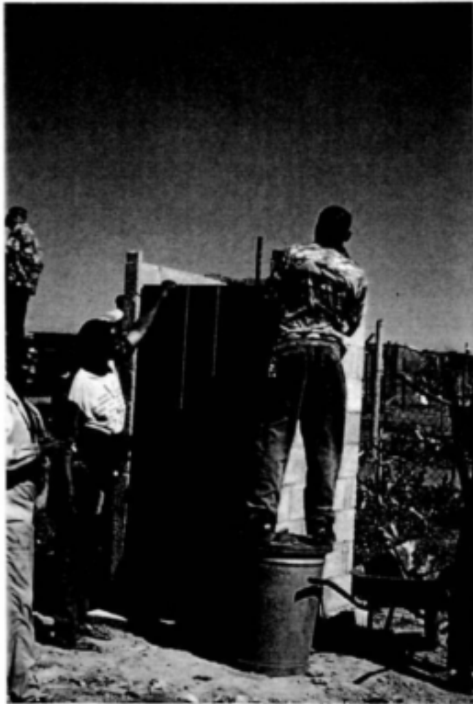
Photograph E : Installation of latrine door prior to positioning of roof slab
