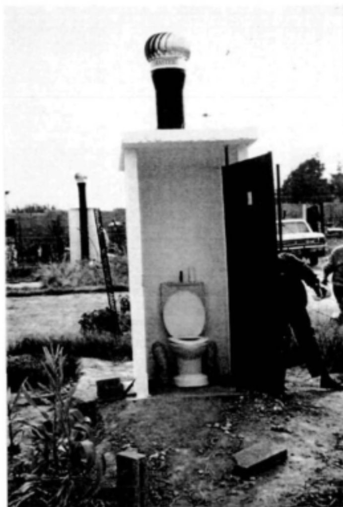
Photograph G : Final finishing of installed Enviro Loo latrine
