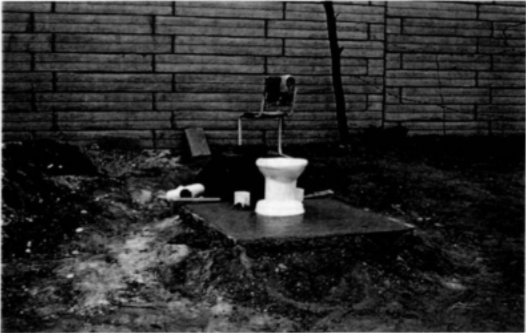
Photograph C : Freshly cast floor slab with toilet bowl in place
