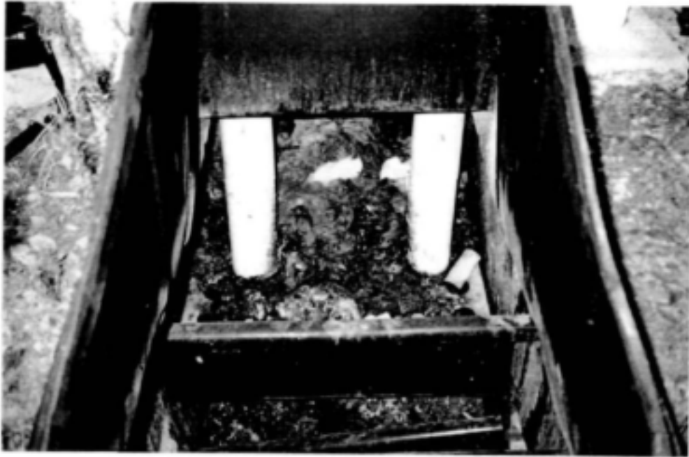
Photograph K : View of typical waste pile in Enviro Loo latrine container (June 1997)
