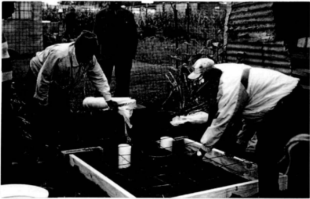
Photograph A : Installation of Enviro Loo latrine in the ground prior to casting of floor slab
