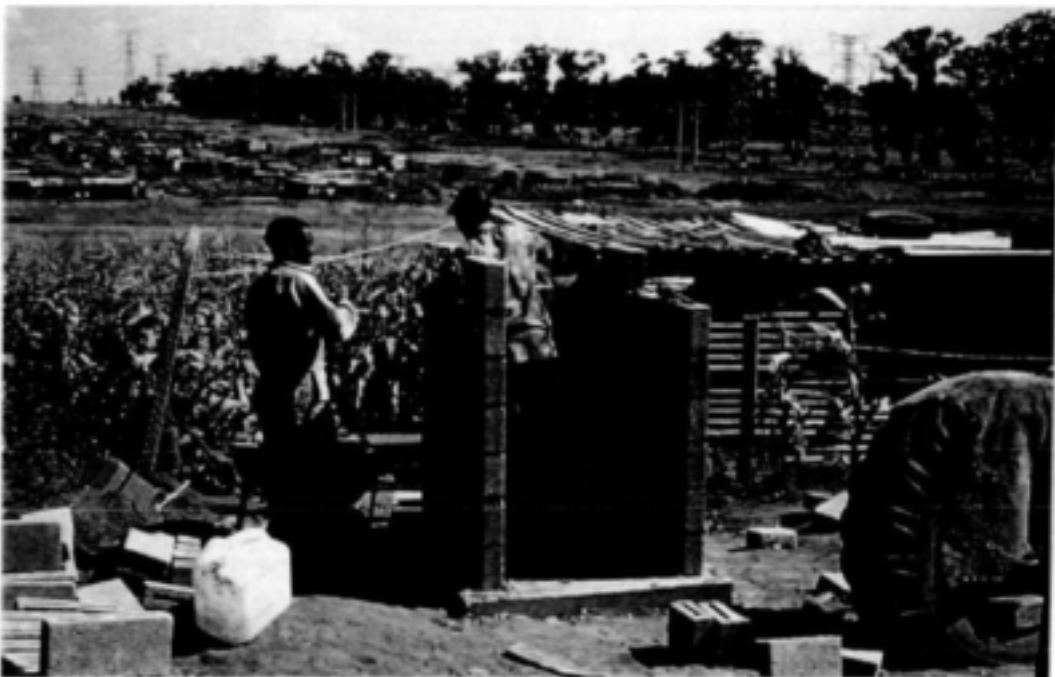
Photograph D : Construction of the walls of the superstructure
