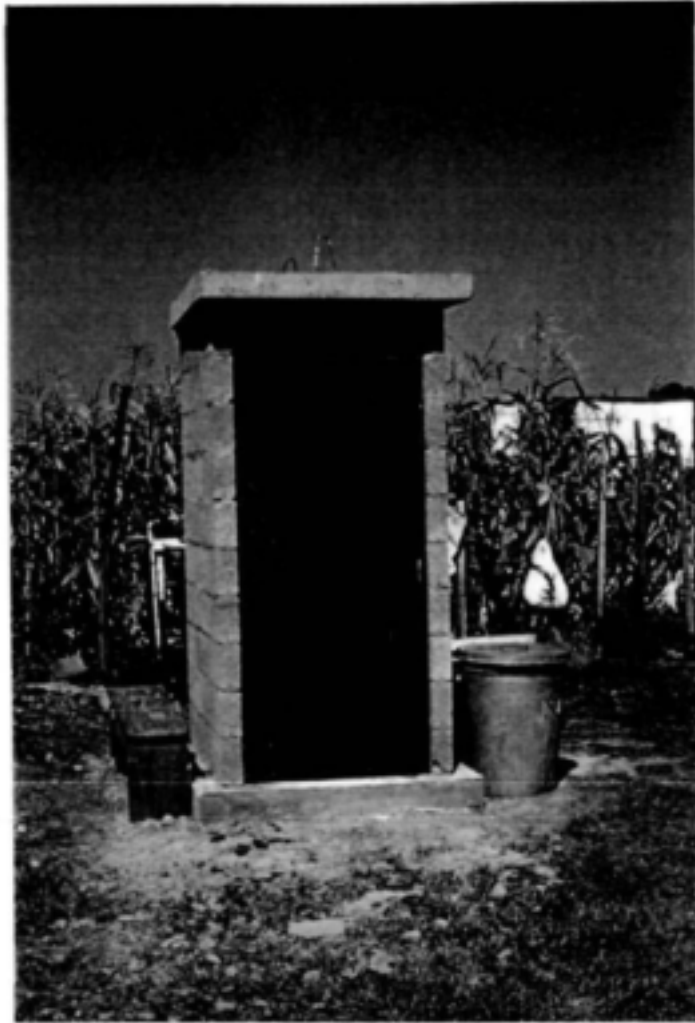
Photograph F : Completed superstructure prior to finishing
