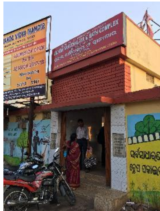
Figure 5: Public Toilet at Badambadi bus stop
