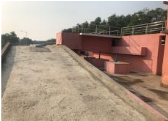
Puri, Odisha STP: (a) Ramp for desludging trucks to go to the receiving chamber (b) Receiving Chamber Photos: Mayank Agrawal, KPMG
