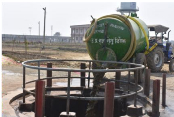
Bingawan, Kanpur STP: Disposal of septage Photos: Shikha Shukla Chhabra
