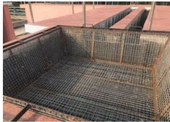
Puri, Odisha STP: (a) Ramp for desludging trucks to go to the receiving chamber (b) Receiving Chamber Photos: Mayank Agrawal, KPMG
