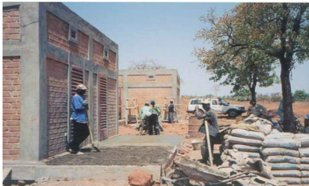
Figure VII-19 and Figure VII-20: The connections between ponds are open to enable easy maintenance and cleaning (left) and two buildings are present on site, one for storage, the other for the technician's office and guardian lodging (right). These buildings were constructed with dirt excavated during construction.
