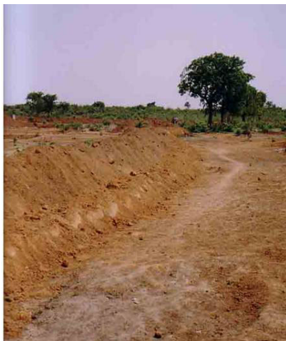
Figure VII-14 (top) and Figure VII-15 (bottom): Another effect of the rainy season: runoff from surrounding land (the ponds sit right on the runoff slope) filled the facultative ponds in June, 2003, necessitating the supplemental building of a reinforced dike wall with bags of compacted dirt
