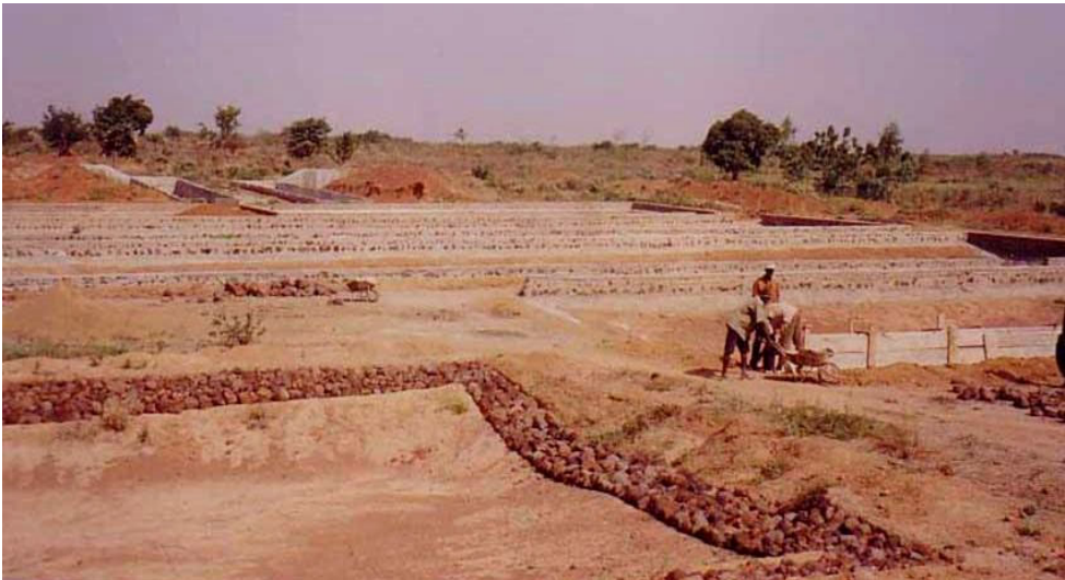
Figure VII-16 and Figure VII-17: (Left) Long view of one settling tank nearing completion, with the second parallel tank visible to the left side. A baffle across the width of the tank prevents short circuiting. (Right) One of two equally sized facultative ponds, with foundation bank stabilization near completion.
