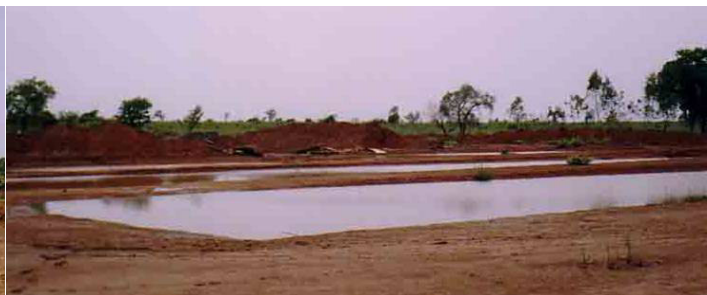
Figure VII-14 (top) and Figure VII-15 (bottom): Another effect of the rainy season: runoff from surrounding land (the ponds sit right on the runoff slope) filled the facultative ponds in June, 2003, necessitating the supplemental building of a reinforced dike wall with bags of compacted dirt
