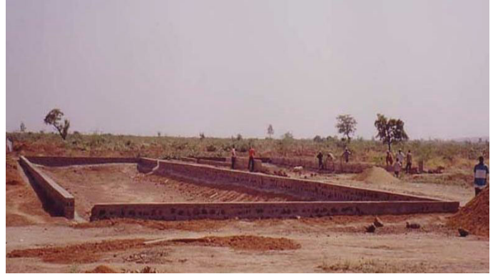
Figure VII-16 and Figure VII-17: (Left) Long view of one settling tank nearing completion, with the second parallel tank visible to the left side. A baffle across the width of the tank prevents short circuiting. (Right) One of two equally sized facultative ponds, with foundation bank stabilization near completion.
