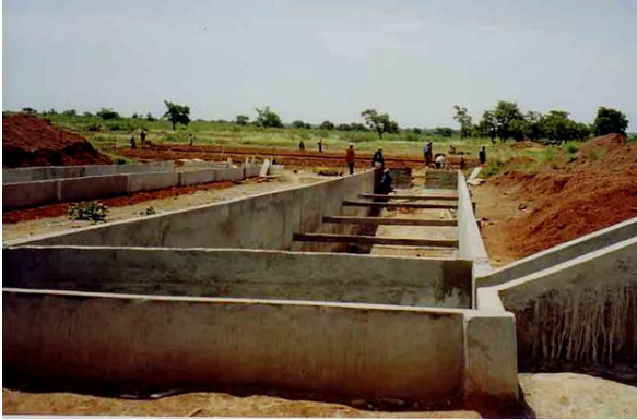
Figure VII-16 and Figure VII-17: (Left) Long view of one settling tank nearing completion, with the second parallel tank visible to the left side. A baffle across the width of the tank prevents short circuiting. (Right) One of two equally sized facultative ponds, with foundation bank stabilization near completion.
