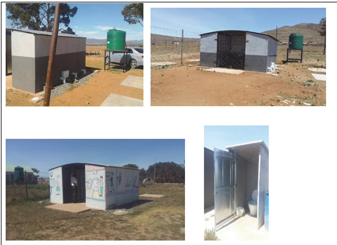
Fig13: Examples of EC school toilet blocks – all in good condition and well-looked after
