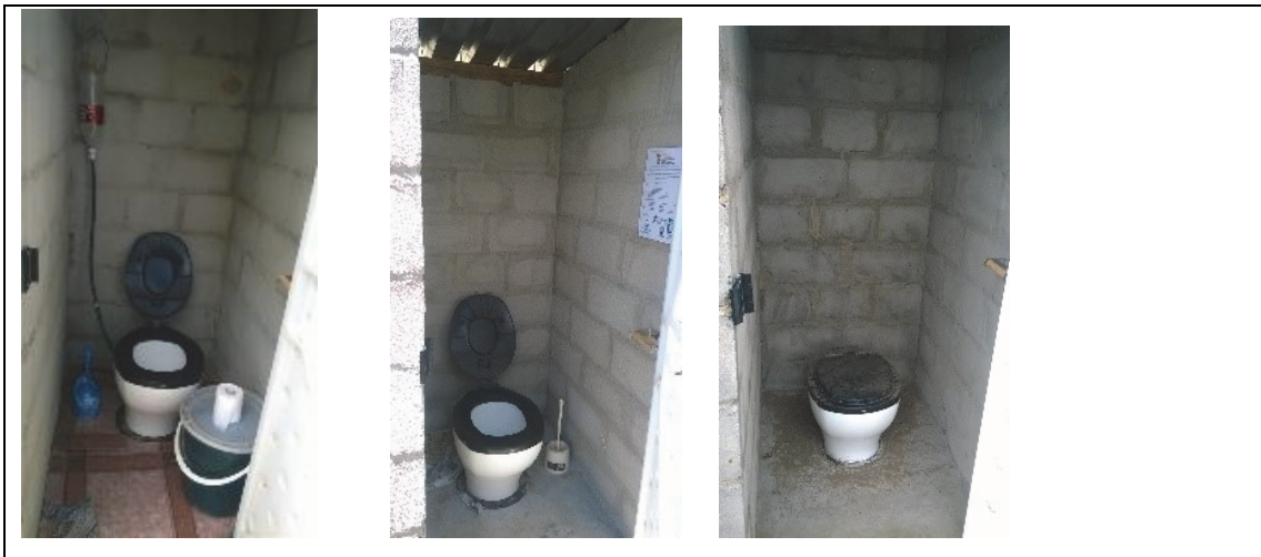
Fig14: Examples of Amajuba household toilets inspected
