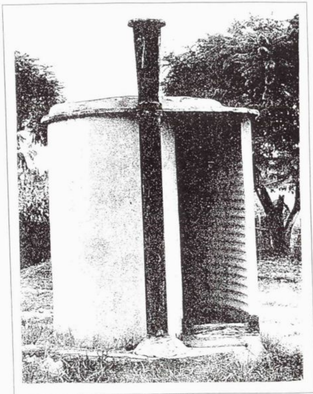
Figure 7.6: Photo of the ferrocement spiral VIP toilet in Zimbabwe
