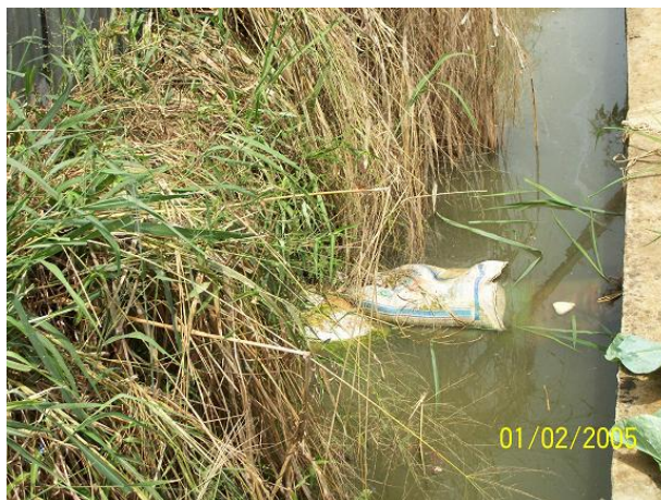
Picture 8: New dam in Network 4's drain
