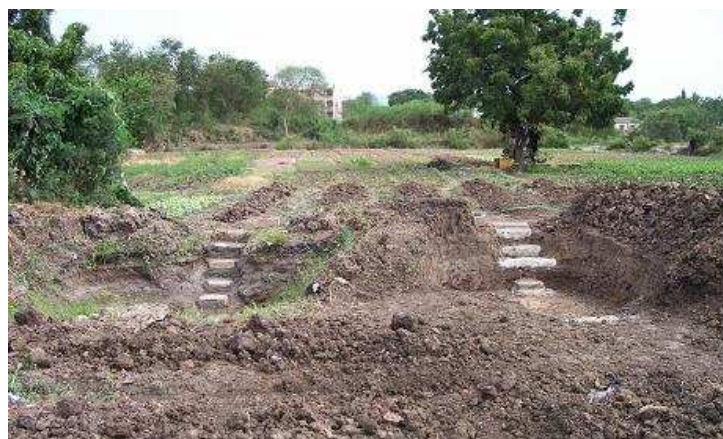
Picture 7: Two individual ponds next to each other
