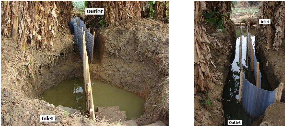
Picture 4: Baffles and plug flow retention pond in Network 4
