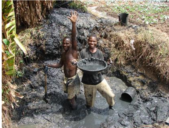
Picture 10: Removal of sediments prior to digging in P3-N4
