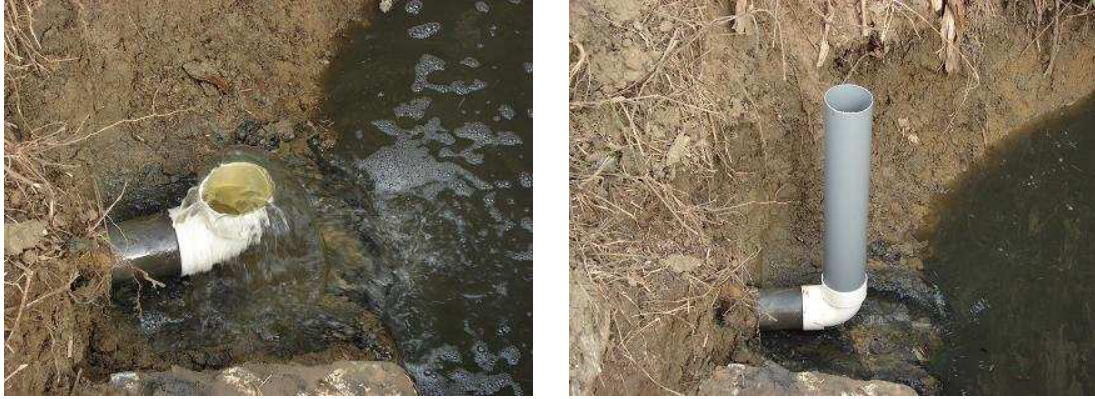
Picture 3: Pipe-elbow floodgate system in Network 4
