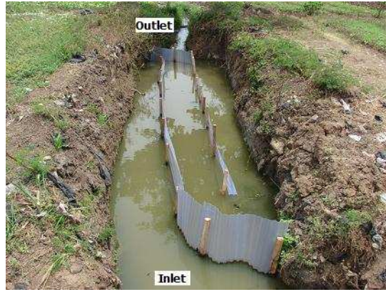
Picture 2: Plug flow retention pond in Network 1
