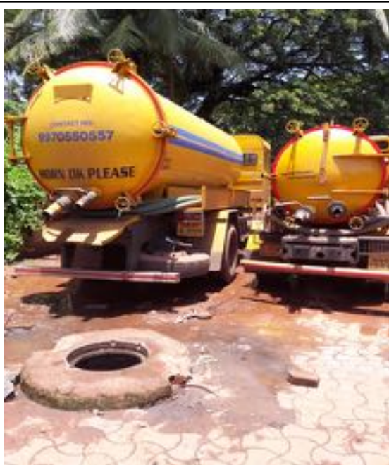
Manhole created for discharge of Septage
