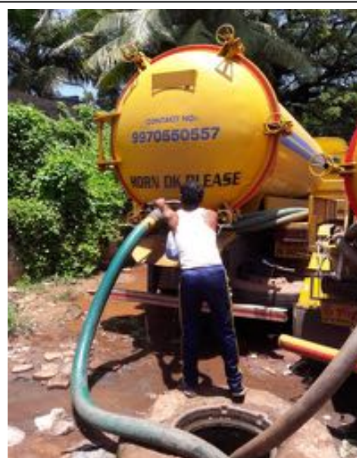
A truck decanting at the manhole
