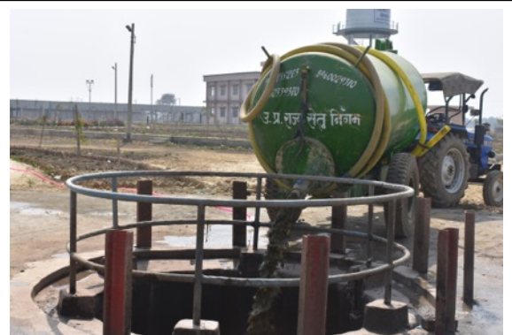
Decanting of Septage in progress at Bingawan STP
