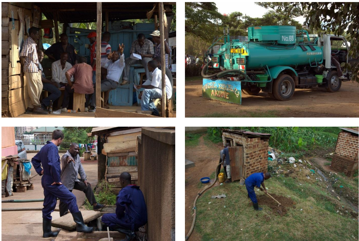
Figure 6: Mechanical faecal sludge emptying service provision. Top left: Members of the PEA. Top right: Vacuum truck. Bottom left: Emptying of septic tank. Bottom right: Emptying of pit latrine (Schoebitz, 2016).
