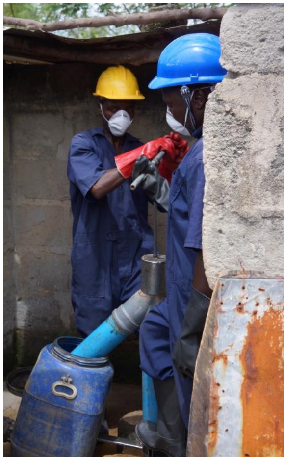
FS emptying with the gulper technology. Photo credit: Moritz Gold
