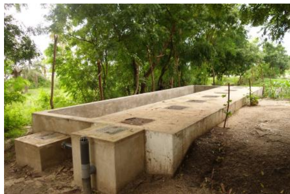
Anaerobic baffled reactor. Photo credit: Imanol Zabaleta
