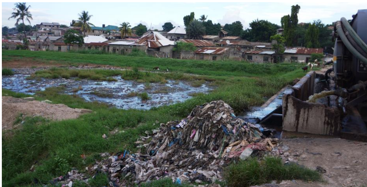
FS disposal by vacuum trucks. Photo credit: Moritz Gold
