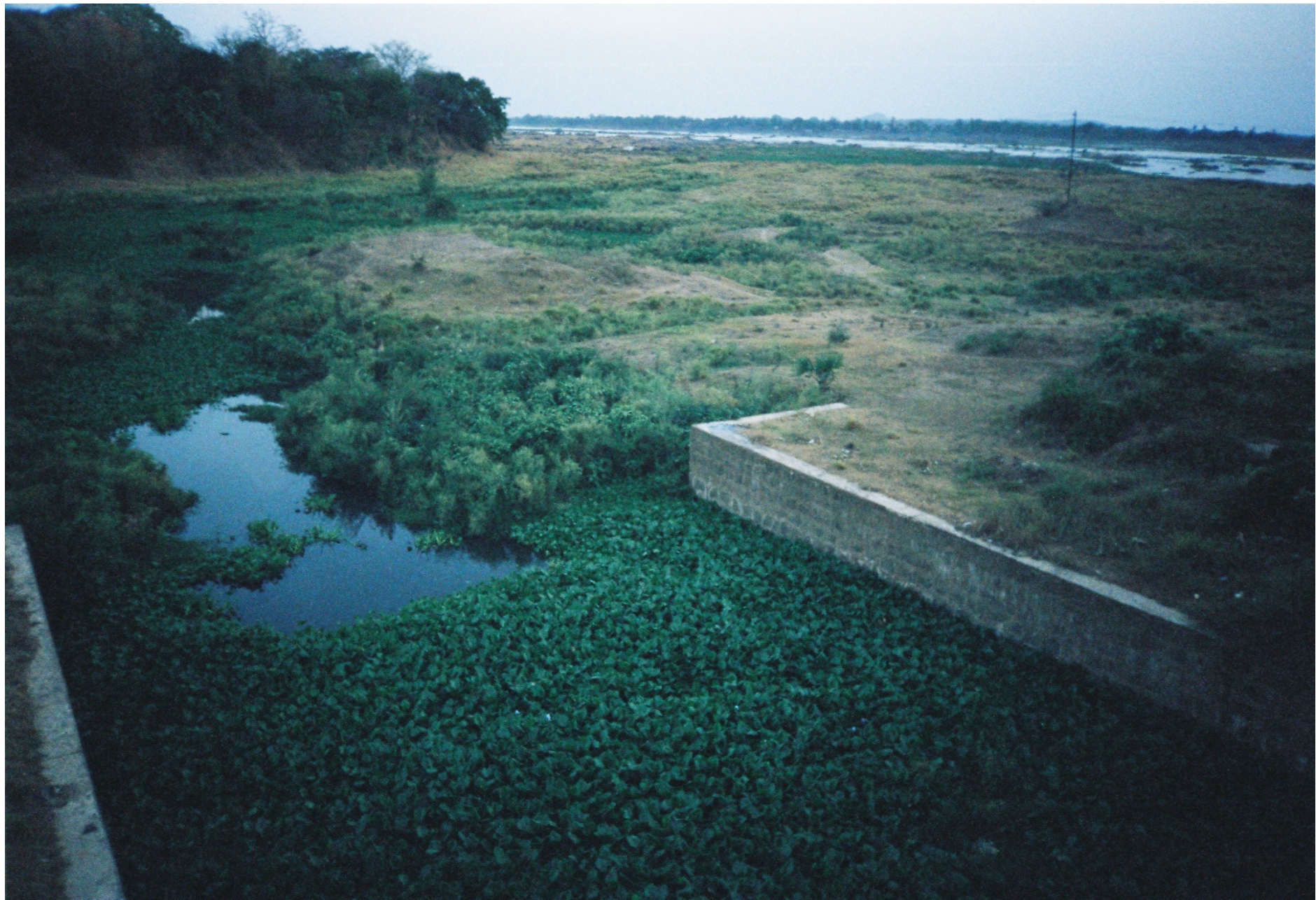
Municipal Drain of Sambalpur Town
