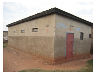
Abandoned Community Toilet
