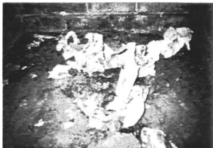
Figure 7. An example of the congested pit latrines
