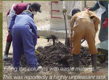
Construction of the concrete columns
