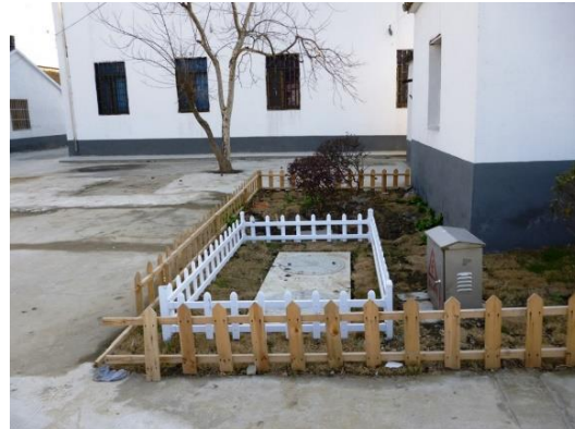
Figure 27. A PAWTP after installation
