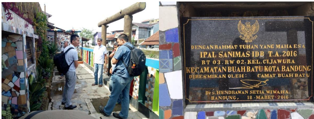
Figure 8. Example of anaerobic type DEWATS system (SANIMAS) installed and managed by a
