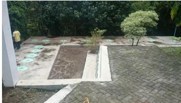
Figure 15. SANIMAS system in Yogyakarta (Source: JSC)
