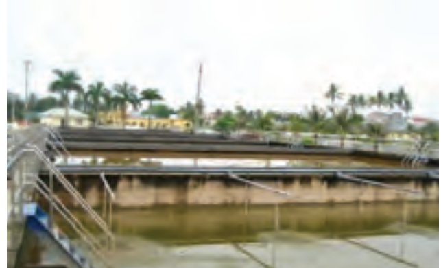
Sludge drying bed at WTP
