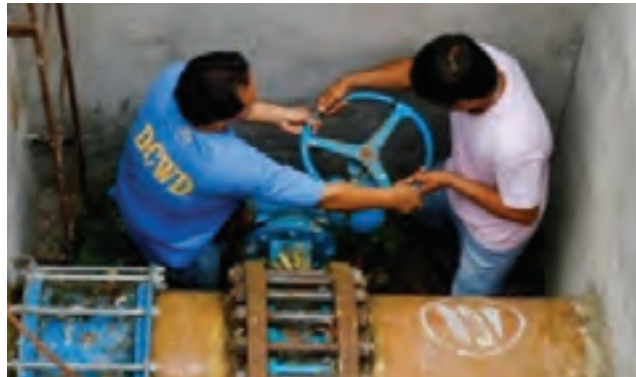
Valve turning for distribution
