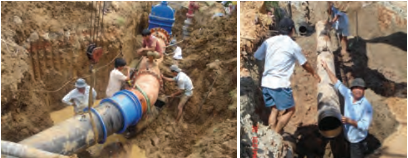
Constructing new transmission pipeline
