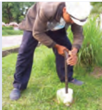
Valve turning for control of distribution
