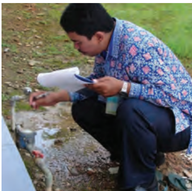
Reading the water pressure
