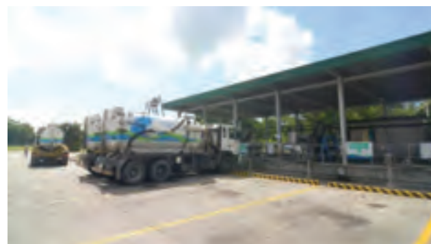
Septage treatment plant
