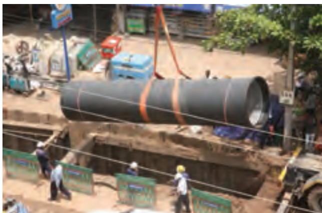
Daytime construction of transmission mains
