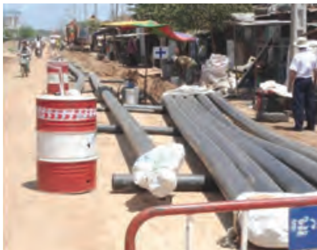
Laying 220 mm high-density polyethylene pipes
