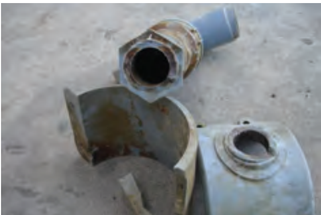
Broken collar on pipe
