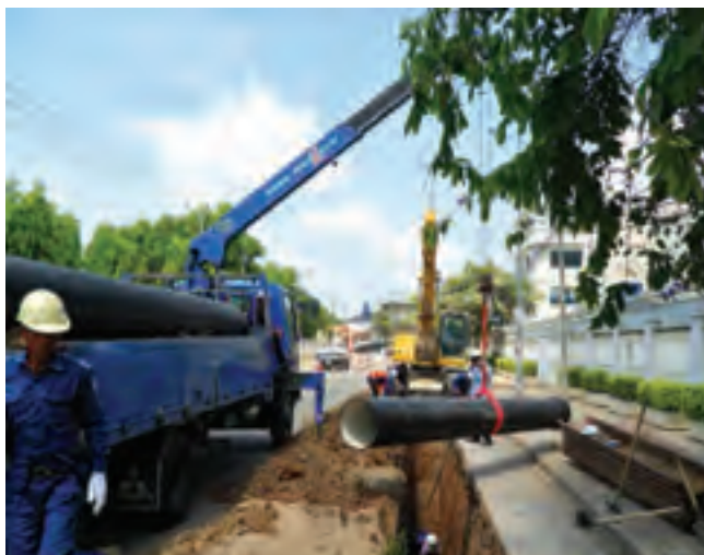
Laying 220 mm high-density polyethylene pipes
