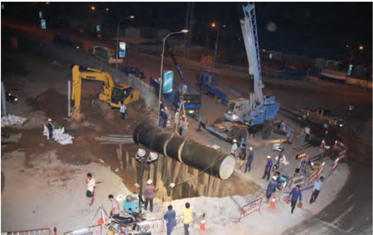
Night-time construction of transmission mains
