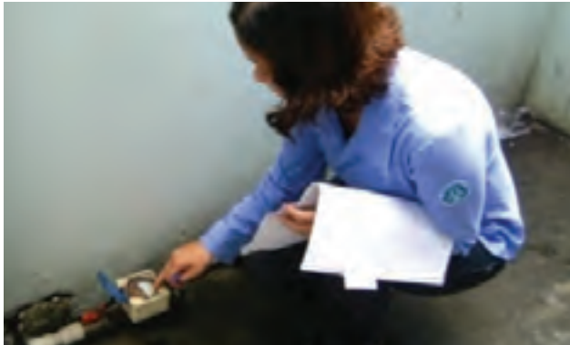
Reading the water meter
