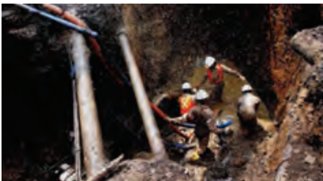
Repairing a distribution leak (c): not easy at great depth
