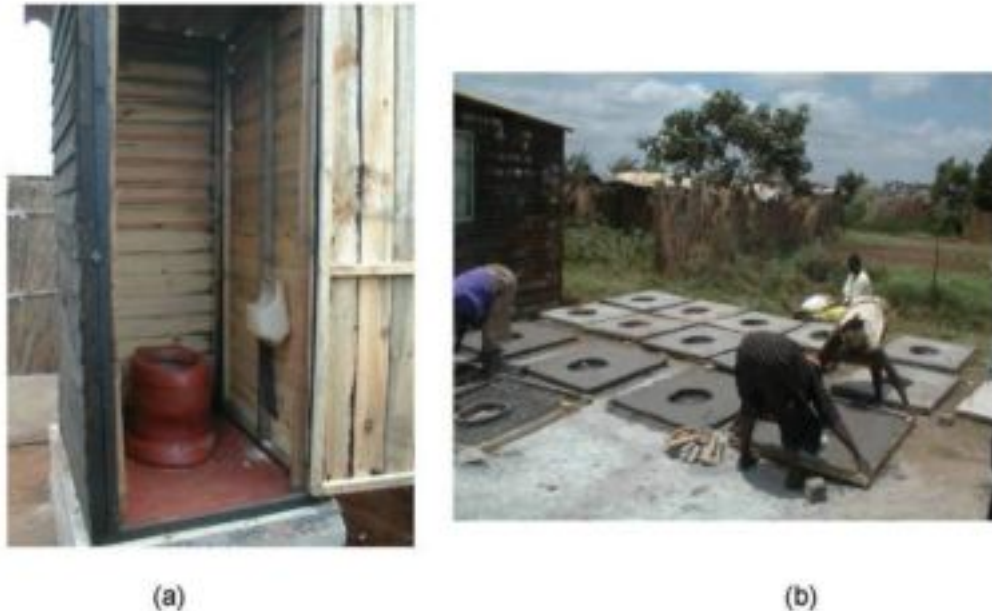
Figure 2.11: Urine-diversion toilets in Zimbabwe.
