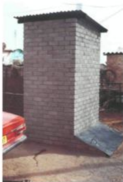
Figure 2.19: Toilets in Hanover, Northern Cape, are constructed with alternating drop-holes for the pedestal, but with a single vault (Photographs: CSIR)
