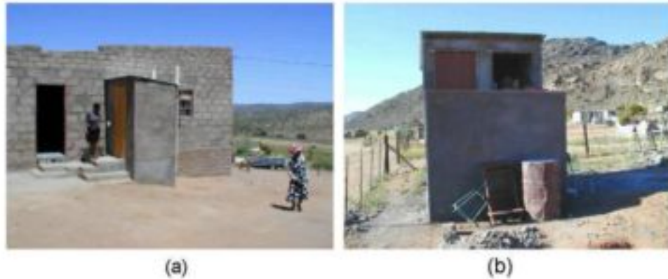
Figure 2.14: Double chamber urine-diversion toilets in Spoegrivier, Northern Cape. (a) Toilet added onto house; (b) separate toilet structure.
