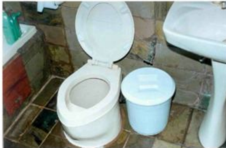
Figure 2.23: Retrofitted urine-diversion toilet in Richard Holden's house in Bellevue, Johannesburg (Photograph: CSIR)
