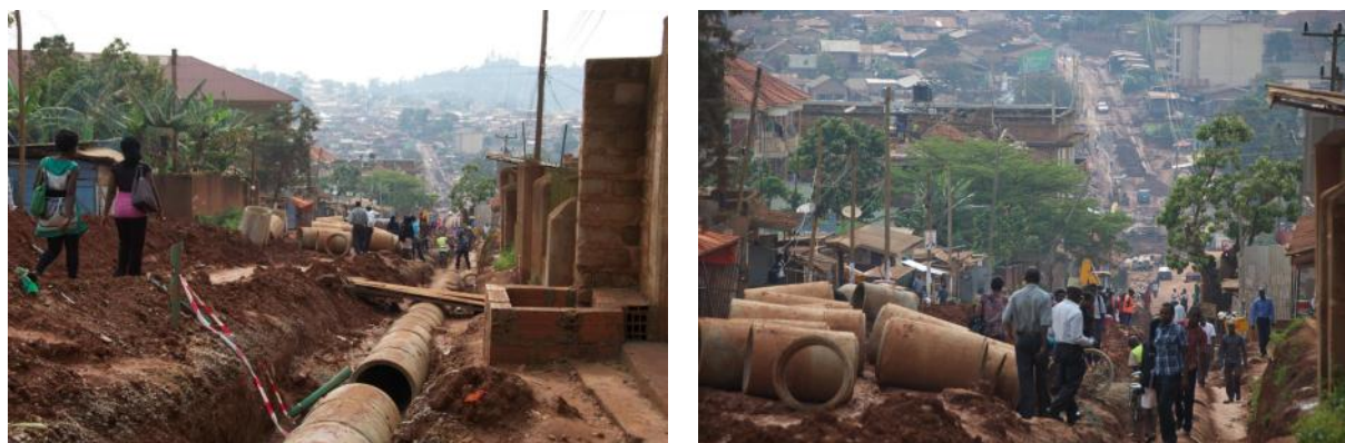
Figure 17: Construction of sewer lines in Kampala. November 2013. Photo credit: Lars Schoebitz
