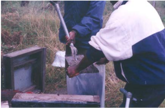
Picture 22: Human excreta being removed from vault in Mthatha (EC)
