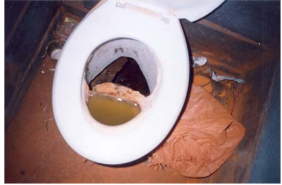
Picture 25: Results of blocked urine pipes in a UD toilet in Augrabies (NC)
