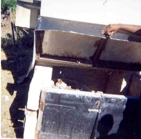
Picture 24: Dry contents in vault of UD toilet (Mthatha) in Eastern Cape
