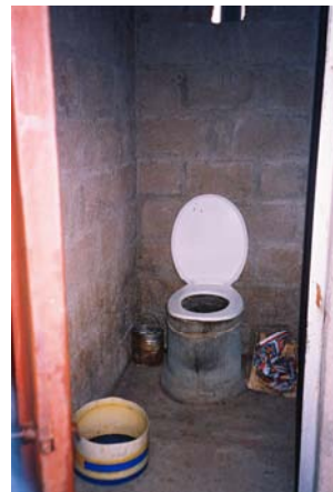
Picture 7: Inside of UD toilet in Augrabies (NC)
