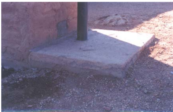
Picture 14: Sealed vault in Augrabies (NC)
