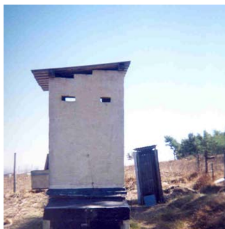
Picture 8: UD toilet in Sinyondweni (Mthatha) with a pit toilet in background
