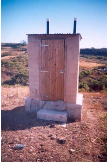
Picture 10: Double vault UD toilet in KZN
