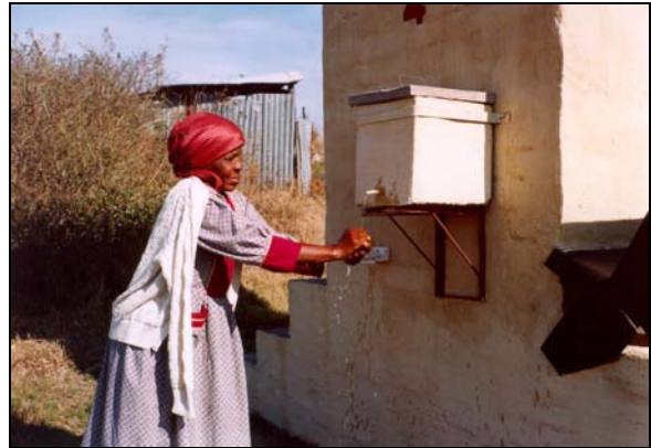
Picture 17: Handwashing facility at a UD toilet in Sinyondweni (Mthatha, EC)
