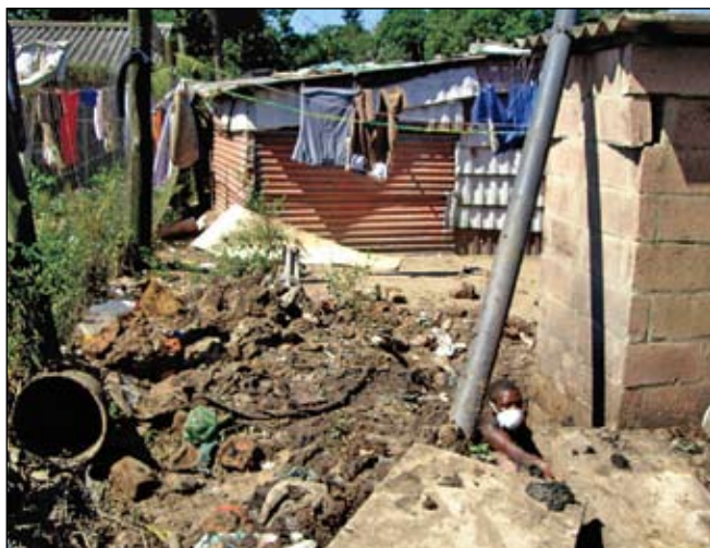
Contents of pit latrines extracted during pit emptying near Tongaat, KwaZulu-Natal.
