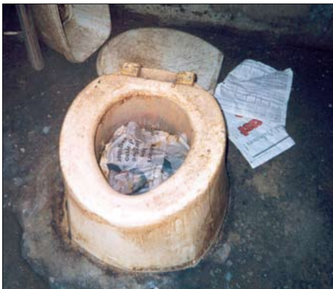
A poorly maintained, overflowing pit latrine, filled with non-biodegradable material.
