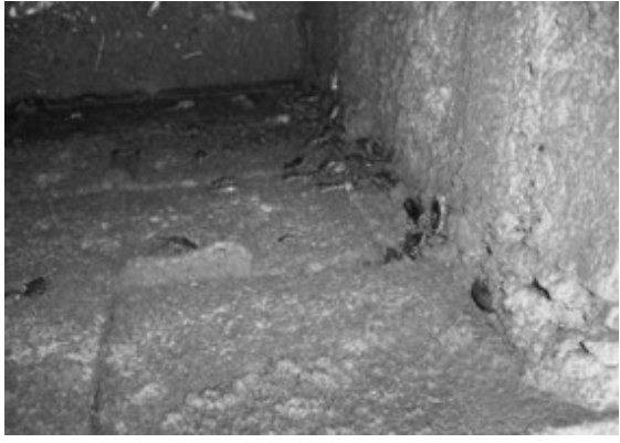
Cockroaches and spiders are regular inhabitants of latrines where the back plate does not fit properly.
