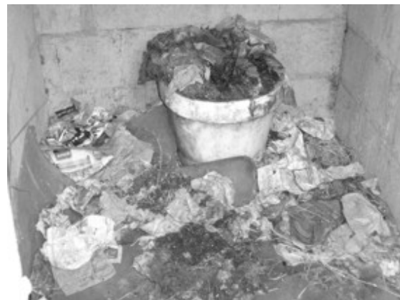
Overflowing pit latrine: the superstructure has become an extension of the pit.
