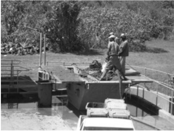
Workers engaged in spraying solids through grid. Note accumulated solid waste in back left of image.
