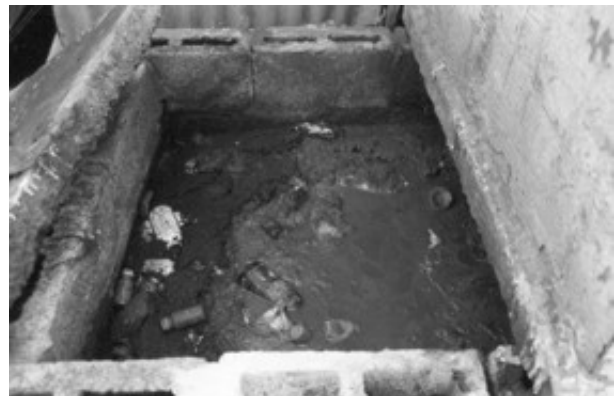
Corresponding pit contents of overflowing VIP latrine viewed through the opened back plate
