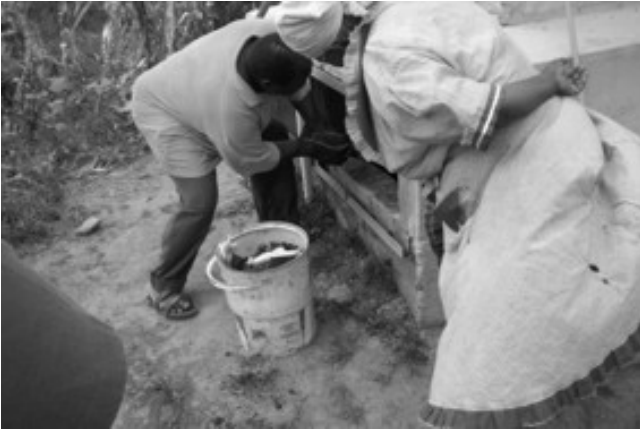
Householders emptying a urine diverting VIP. Householders are encouraged to bury the vault contents on-site.
