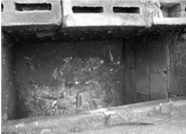
Pit opened for emptying
