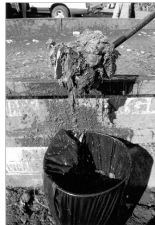
Solid waste transferred to rubbish bags
