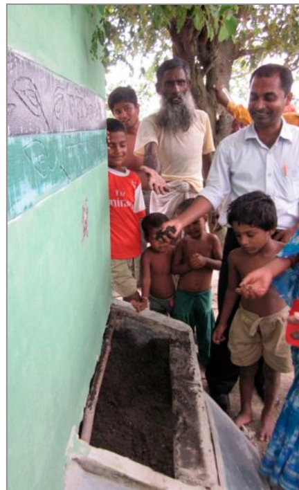
Figure 13: Opening the Feces Chamber Owners of a UDDT in the Amarak village are encouraged to handle fecal soil conditioner by SPACE field staff after opening their feces chamber for the first time. (Photo: A. Guadagni)
