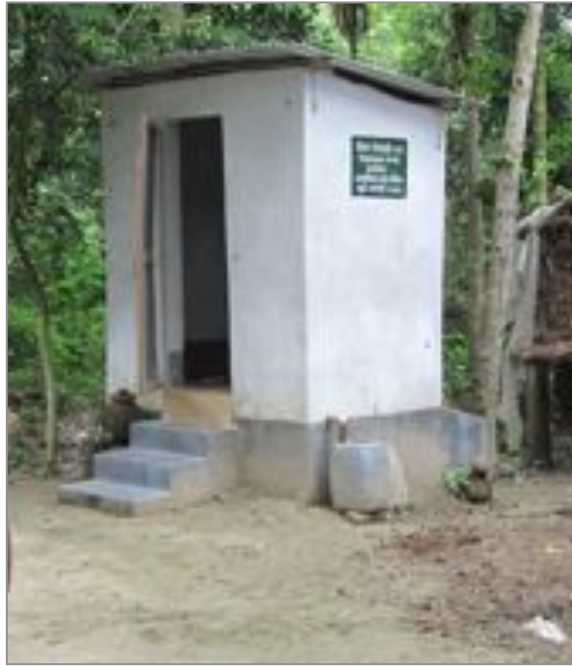
Figure 11: UDDT Super Structure
