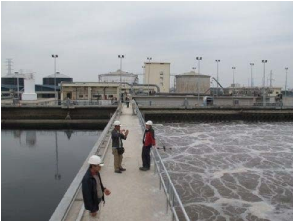
Picture of Yen So WWTP (Nguyen 2015)
