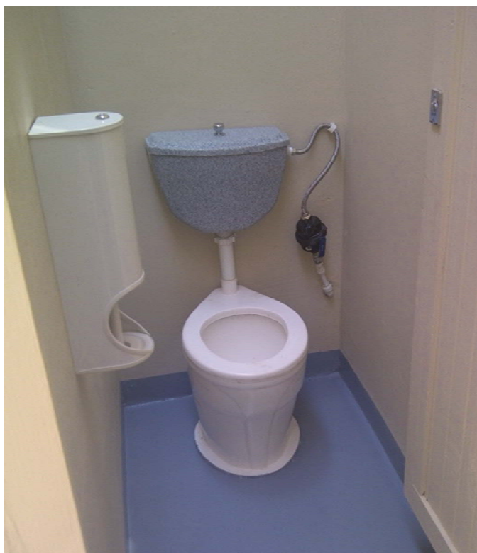
Figure 27: Low flush toilet tested in schools in KwaZulu-Natal
