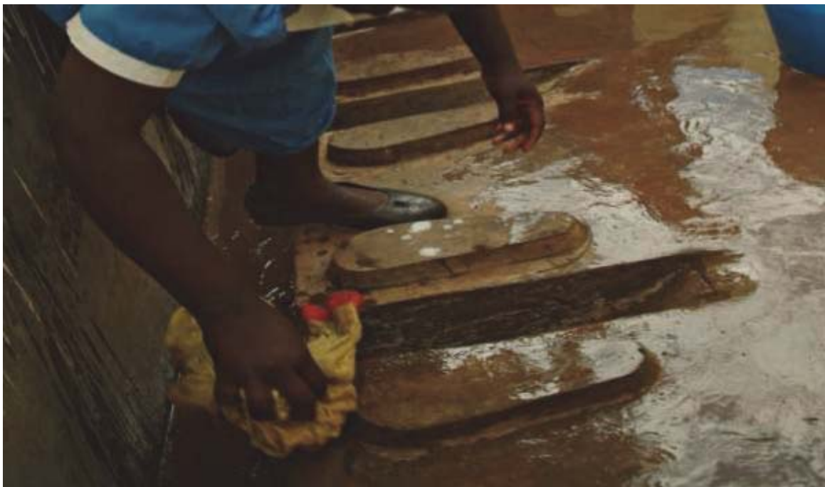
Figure 9: A female urinal design used in schools in Malawi 31
