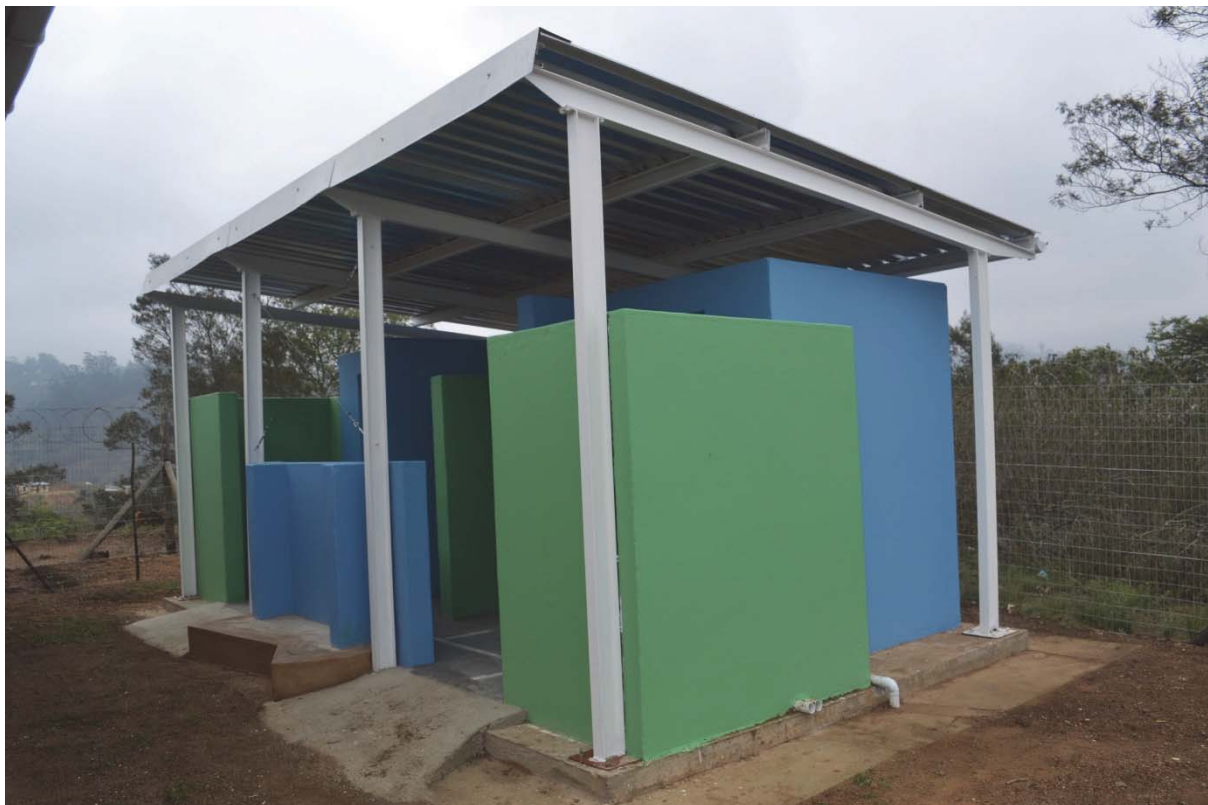
Figure 17: Pour flush sanitation facilities built by LIMA and Save the Children for a crèche
