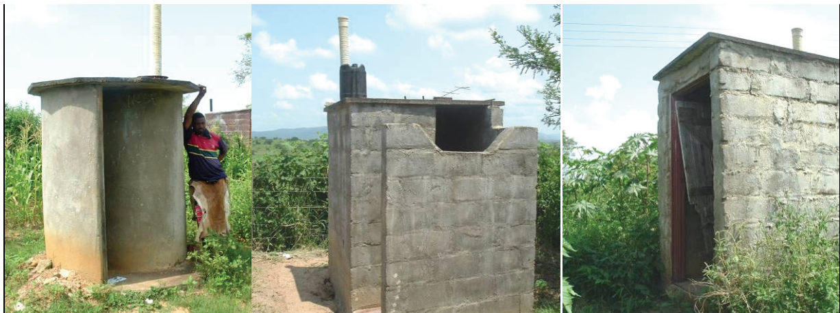
Figure 23: The three types of VIP built in Nkomazi in 1995: spiral mould (left), blocks with no door (centre) and blocks with door (right)
