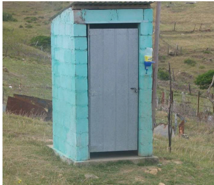
Figure 21: VIP superstructure constructed at Newlands
