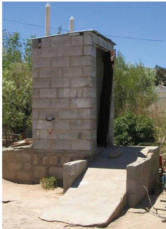
Figure 33: Double urine diversion system, with ramp, at Kammiesberg, Northern Cape
