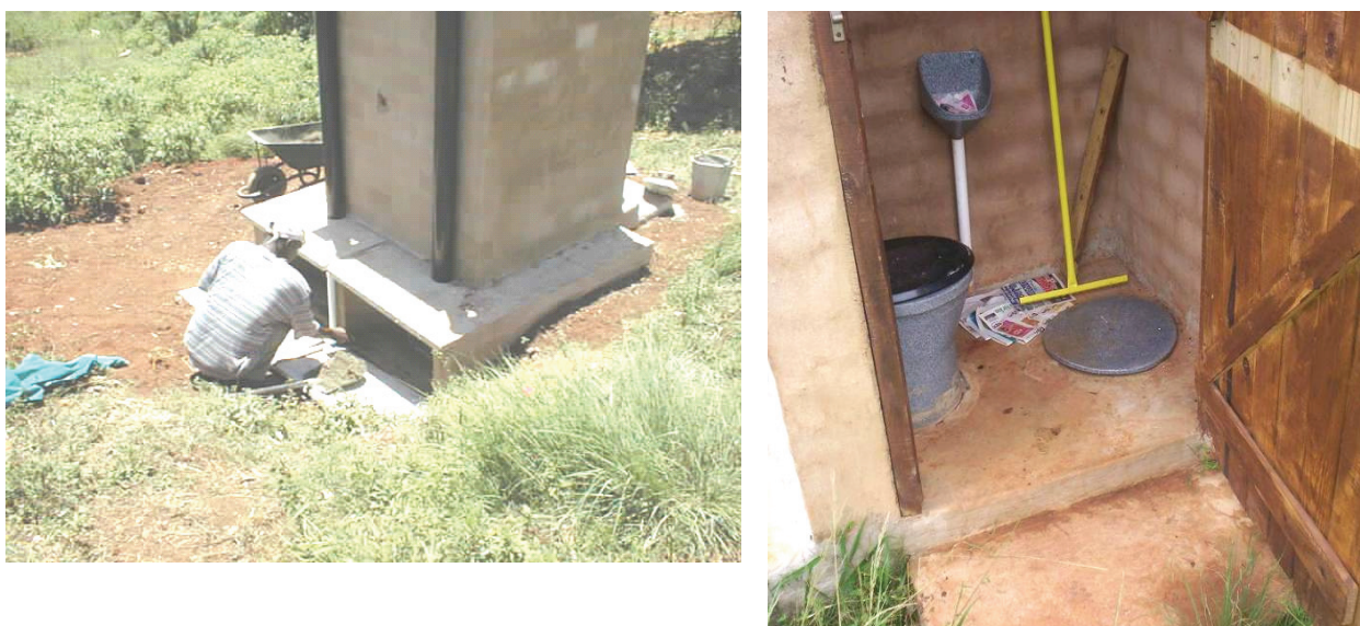
Figure 26: Outside and inside views of the eThekwini double pit Urine Diversion toilet
