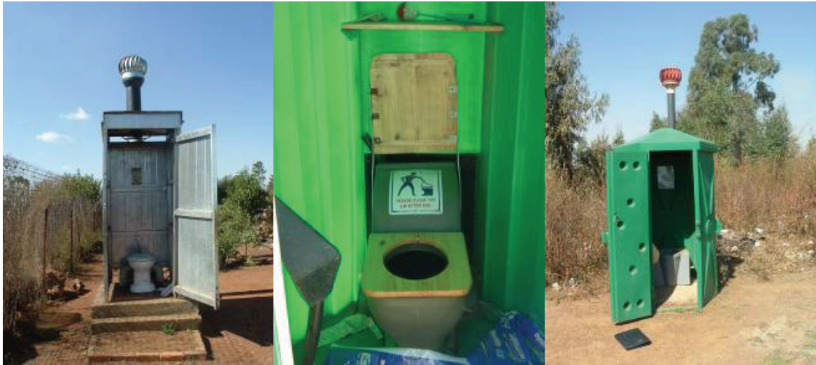
Figure 35: Inside of the superstructures: Enviroloo (left), EcoSan (centre) and SolarSan (right)
