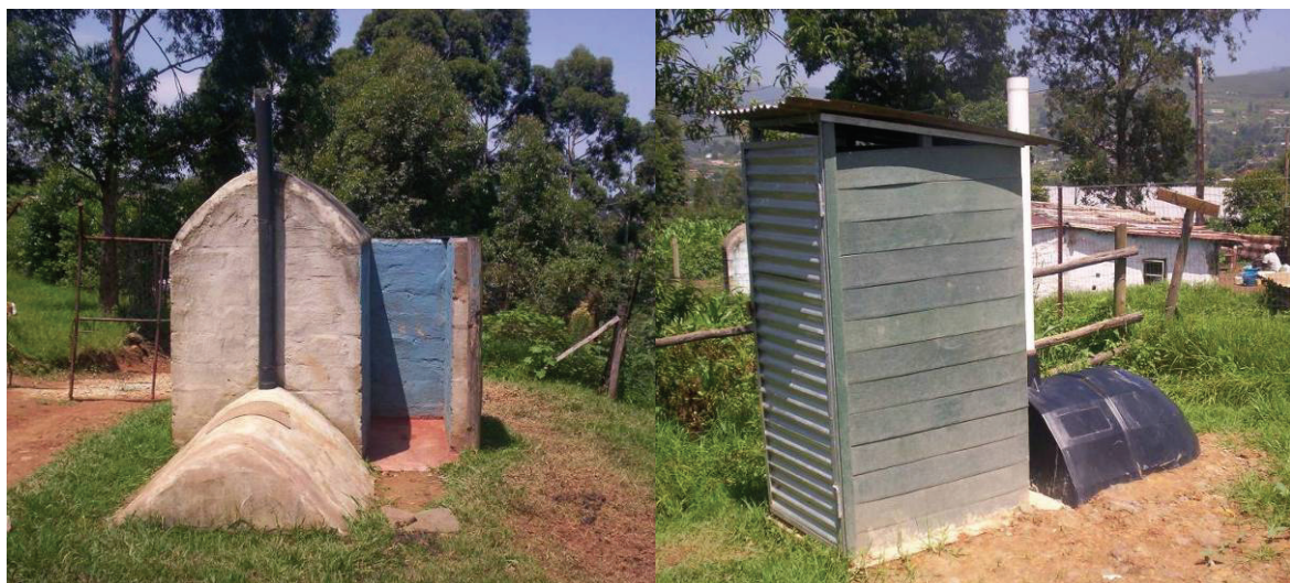
Figure 18: Phungalutho latrine constructed in Inadi in 1995, photo taken in 2006; new VIP (PET calcamite) with a movable superstructure that some families have had constructed when the Phungalutho latrine built in 1995 became full
