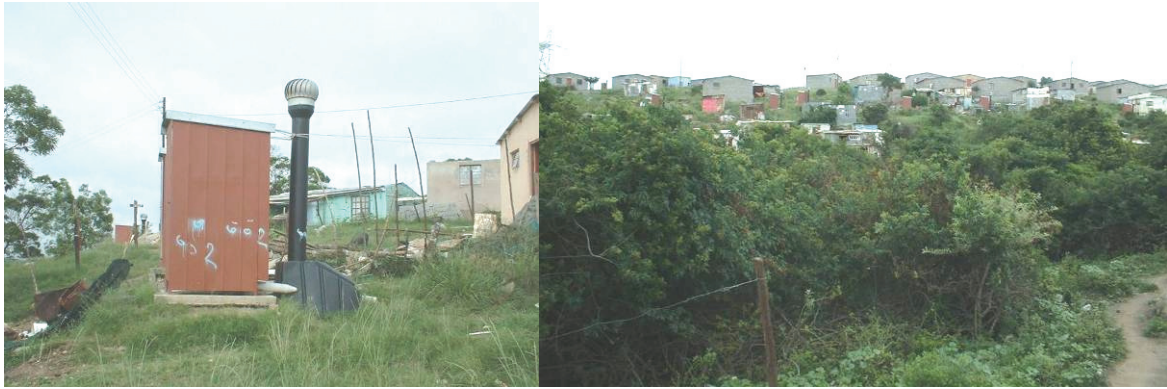
Figure 29: Enviro Loo (left); valley where residents have disposed of waste from the Enviro Loos (right)
