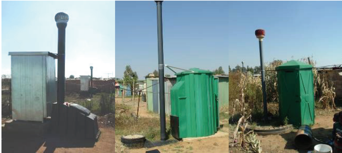
Figure 34: The three dry toilets trialled by Ekurhuleni Metropolitan Municipality: Enviro Loo (left), EcoSan (centre) and SolarSan (right)
