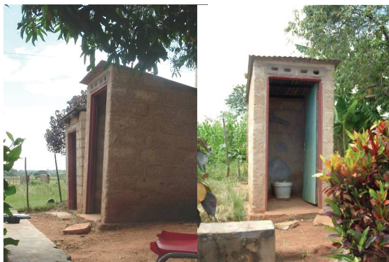
Figure 24: VIP latrines constructed at the Newline sanitation project in 1995
