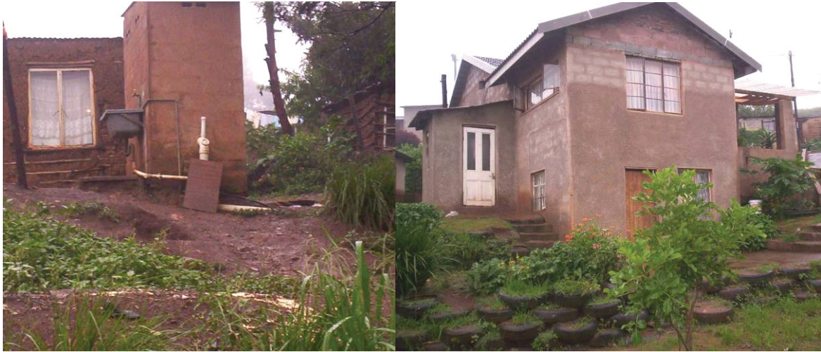
Figure 39: Toilet block for waterborne sanitation at Ntuthukoville (left); toilet block on the left hand side of the building has been incorporated into this house so the toilet is now indoors (right)
