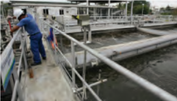
South Septage Treatment Plant (Source: S. Griffiths)
