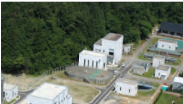
Aerial view of the Suzu City wastewater treatment facility. (Source: Saburo Matsui)
