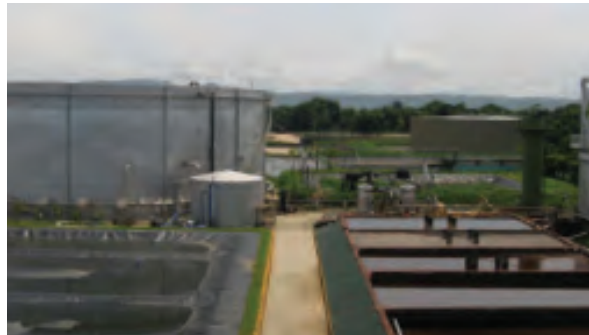
Thermophilic anaerobic digester and lagoons (Source: G. Tee)
