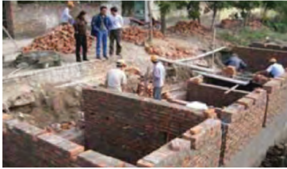
During construction of the anaerobic baffled reactor (Source: ADB)
