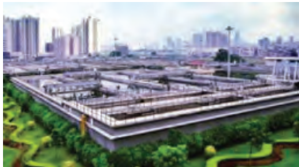
Liede sewage treatment plant (Source: Lin Duan)
