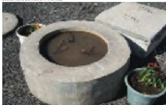
Area of top manhole, above the biogas fixed dome (Source: SuSanA)
