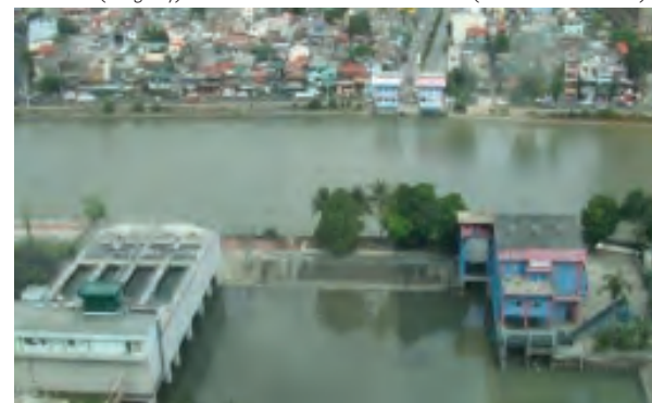
Poblacion STP (Makati City): elevated and on top of a Flood Control Pond (Source: MWCI)
