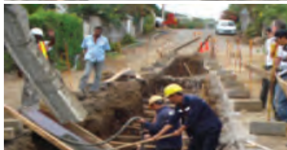
Construction of sewerage system. (Source: IWA)
