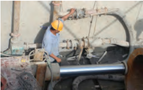
Sewerage construction (Source: ADB)
