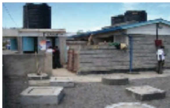
Sanitation facility with water kiosk. Underground biogas plant in front (Source: Sustainable Sanitation Alliance)
