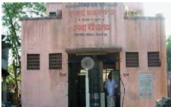
Toilet block (Source: Water and Sanitation Program)
