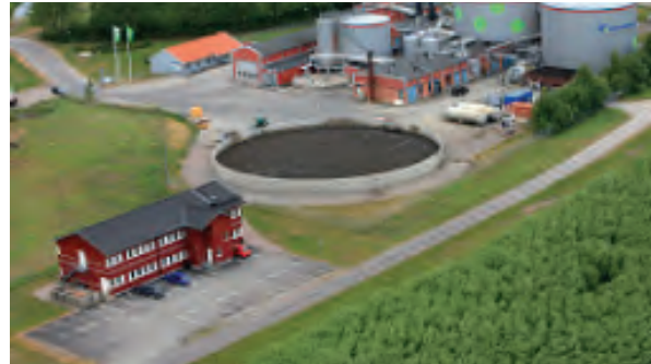
Linköping biogas plant (Source: Svensk Biogas)
