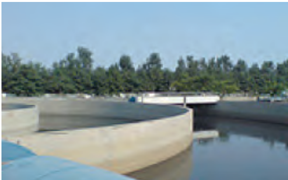
Wastewater treatment plant in Hebei (Source: ADB)
