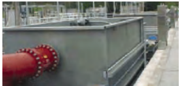
Orange County wastewater treatment plant (Source: IWA)
