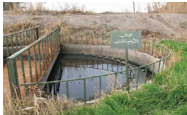
Sedimentation Tank (Source: IWA)
