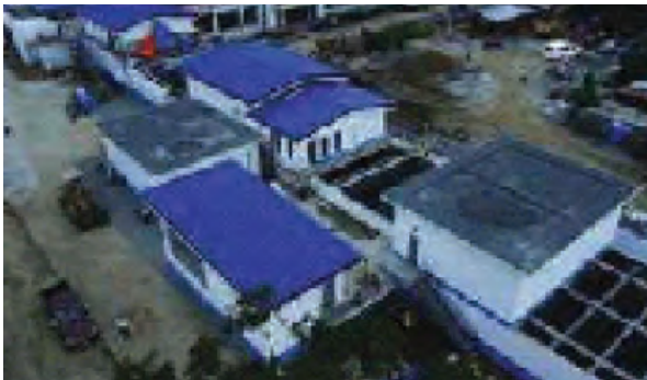
Conventional Activated Sludge (Bahay Toro STP) (Source: MWSI)
