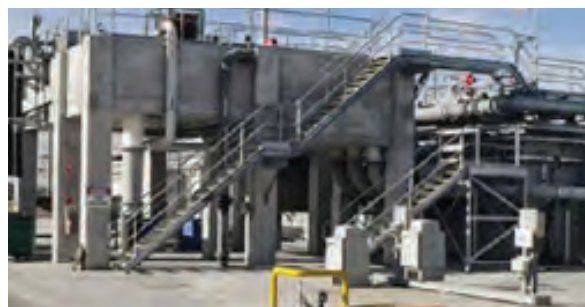
Altona wastewater treatment plant (Source: M. Giesemann)
