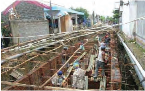
During construction (Source: Yuyun Ismawati)
