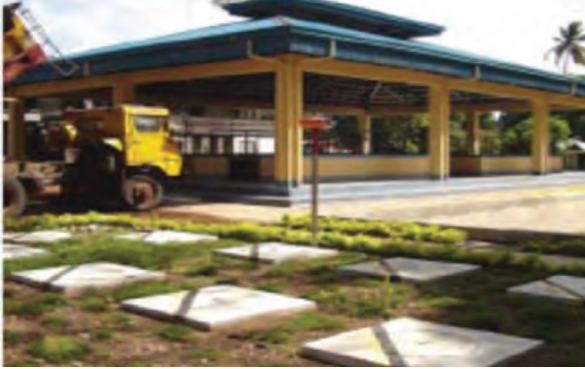
View of the anaerobic treatment modules: settling tank (ST), anaerobic baffled reactor (ABR), and anaerobic filter (AF). (Source: BORDA)
