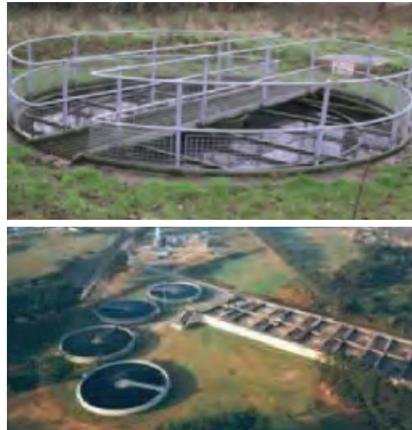
Wastewater treatment plant in Durban (Source: IWA)
