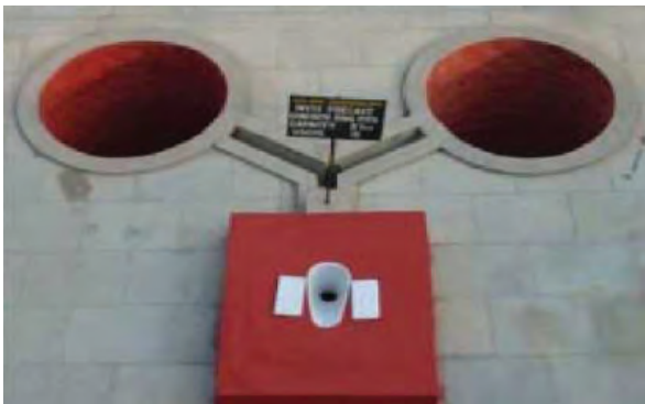
Sulabh Two-Pit-Pour-Flush Toilet (Source: B. Pathak)
