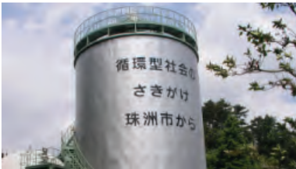
Vertical steel methane fermentation tank. (Source: Saburo Matsui)
