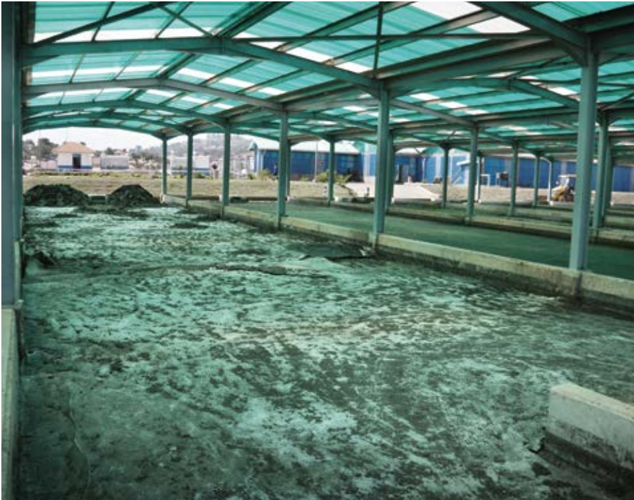
Photo 2: Drying beds at NWSC Lubigi Wastewater and Faecal Sludge Treatment Plant in Kampala, Uganda.
