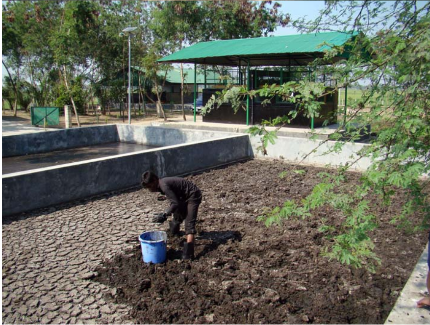
Faecal Sludge Collected by Vaccu-Tug and Discharged in the Drying Bed and later Co-composted with Organic Waste to Produce Compost
